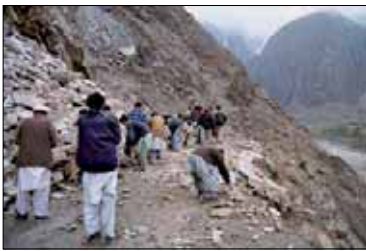
Road blocked — KKH
