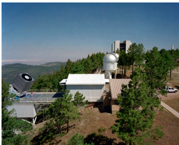
Apache Point Observatorium, USA/New Mexico (5)
